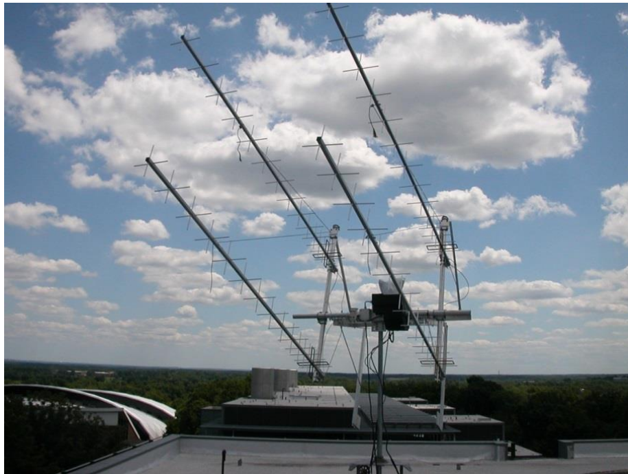
Fig. 7. – The four-Yagi 432 MHz array at W2PU.
